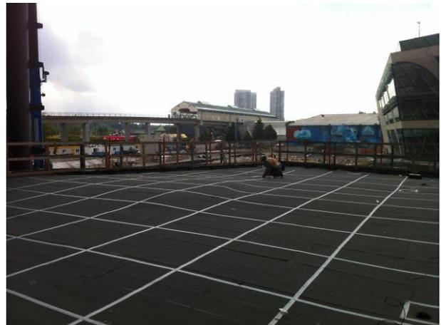
Once a leak has been localized to a gridded area, the conductors can be used to apply a locating signal for the Electric Gradient Leak Locate system (EGLL) to further pin-point any breach location within a grid size area. The leak locate grid system provides an accurate method to monitor and maintain a wide range of covered roof types and sizes and is particularly effective on inverted roofs where the membrane is not easily accessible.
