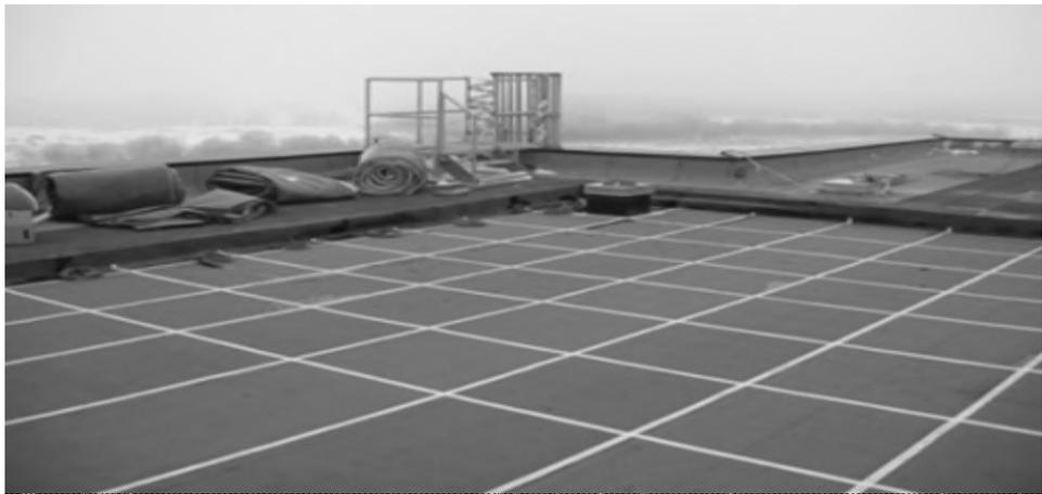
The leakage current level is then mapped out on the as-built grid plan thereby identifying and localizing any leaking sections underneath the membrane. By performing an automated routine leak detection and locate procedure, membrane leaks can be identified and located to an area within a grid section.
